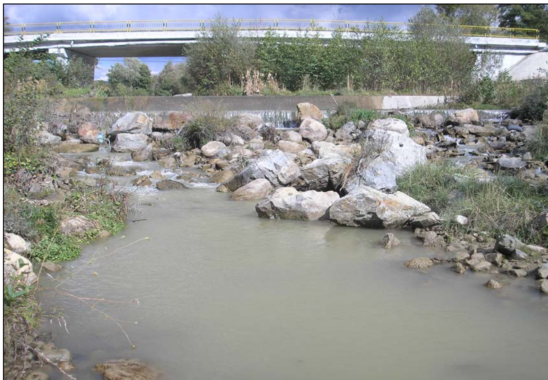
Figure 17: Stone steps which do not permit the fish to migrate.
