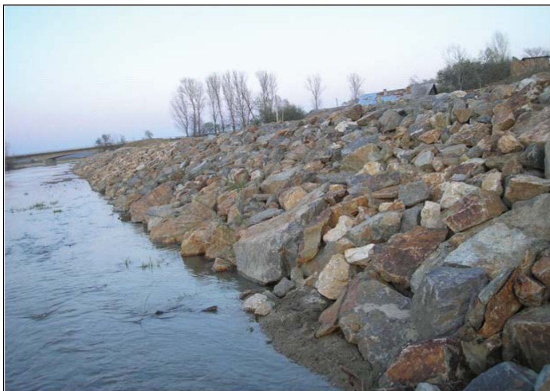
Figure 23: River linearization using rockfill banks; near the Dinculești locality.
