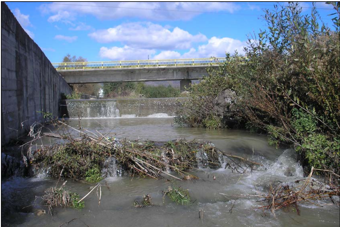
Figure 15: Concrete barrage with no fish leather.
